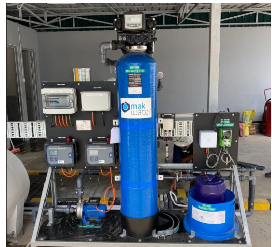
Multimedia filtration (MMF) and hypochlorite disinfection dosing
