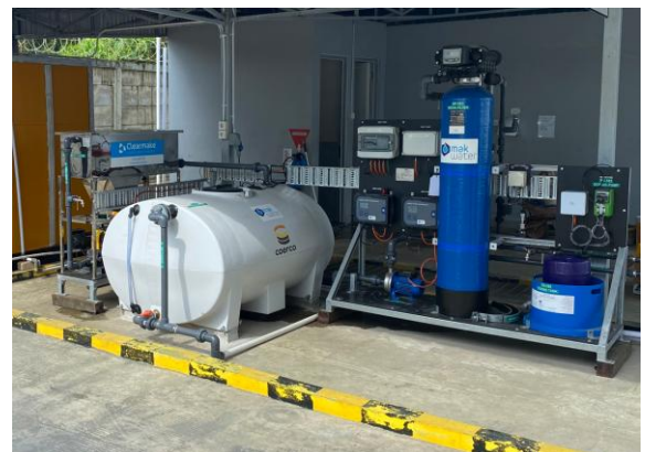
Compact, skid-mounted treatment train
